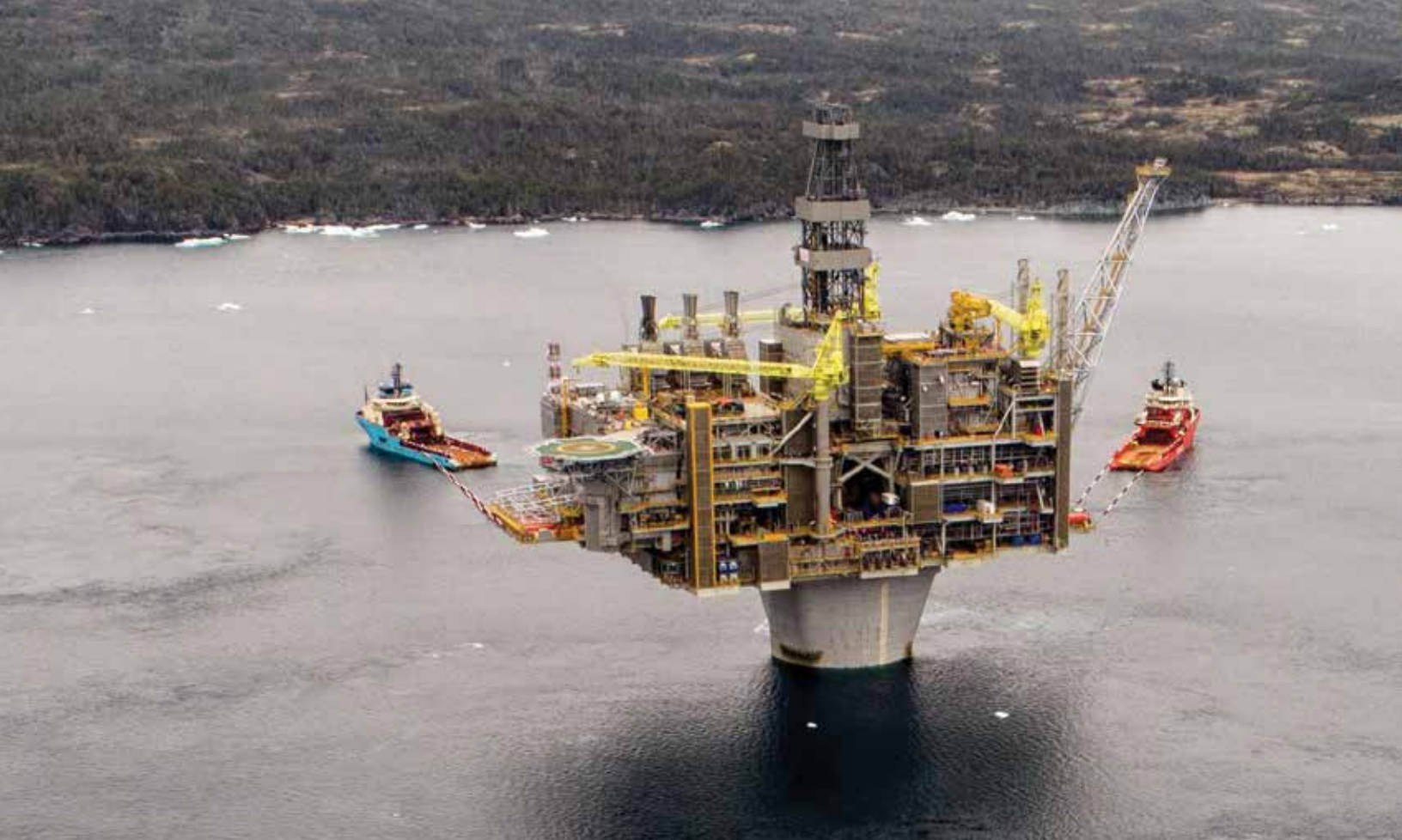
The Hebron GBS departed Bull Arm on June 3 and was installed at its offshore location on June 14. First oil was produced a month ahead of schedule, on November 27.
